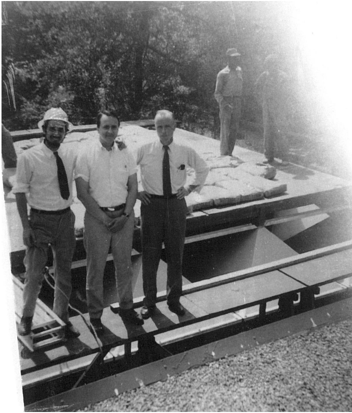
Figure 11. Renzo Piano (left) with Nick Gianopoulos (center) during the load test of the skylight, Philadelphia, 1969. (Fondazione Renzo Piano)
